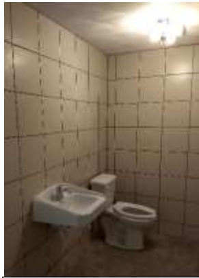
One of two bathrooms nearly completed
