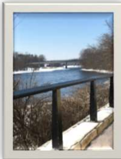
View to the west of the Center Avenue Bridge from the new section of the trail.
